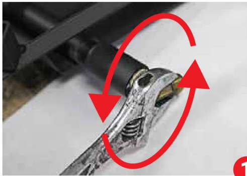
Removal of Natural Gas elbow and orifice
